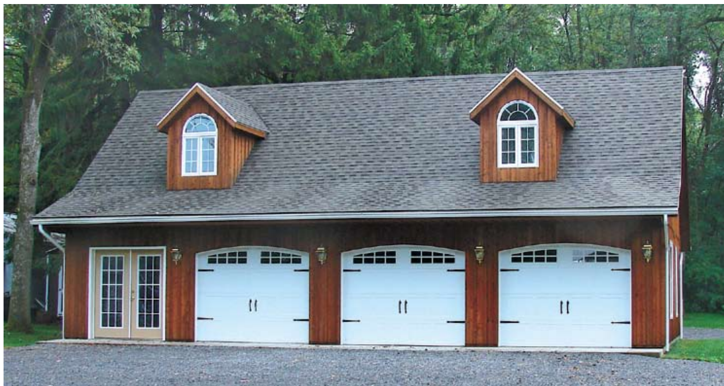
Above right: Builder and old-fashioned craftsman Simon Wickey with the tools of his trade. Above: Larch-sided garage built by Wickey on Keuka Lake’s Marilena Point.
